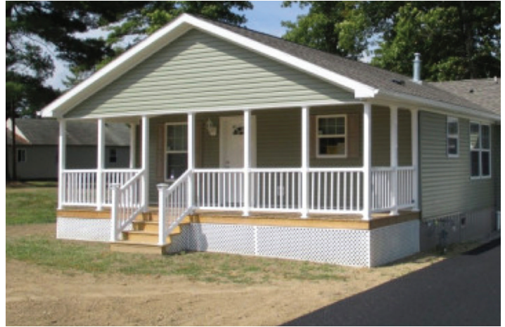
Crawlspace under front end wall, behind lattice work.
