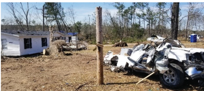
Manufactured home structurally intact, vehicle destroyed (Lee County, Alabama - March 2019).
