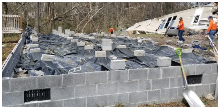
Manufactured home not adequately secured to ground slides off support piers. (Lee County, Alabama - March 2019).
