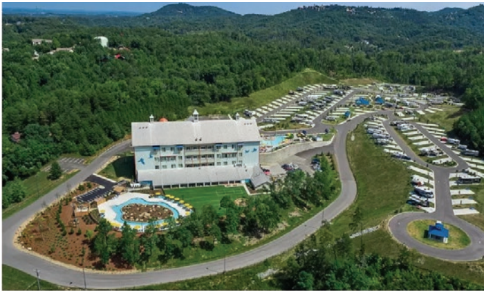
Courtesy of Safe Harbor Development Camp Margaritaville in Pigeon Forge, Tennessee
